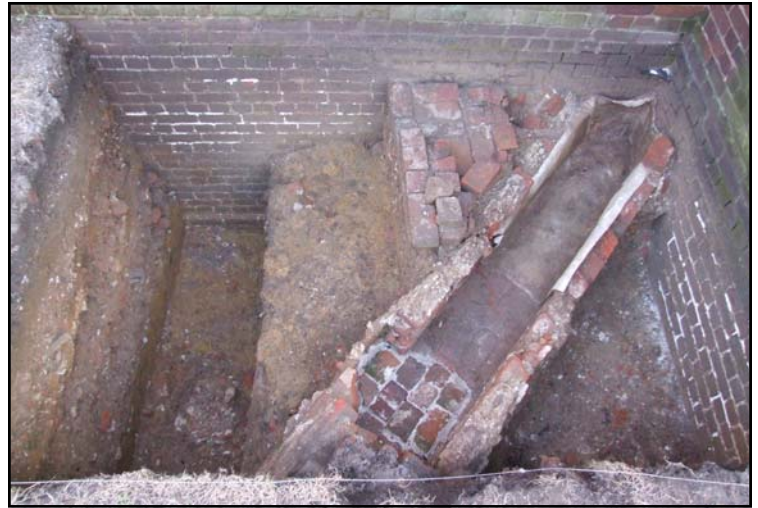
The lead-lined drain in Rosewell's northwest corner.
